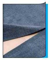
Carpet joints must be carefully butted or double cut and seamed
